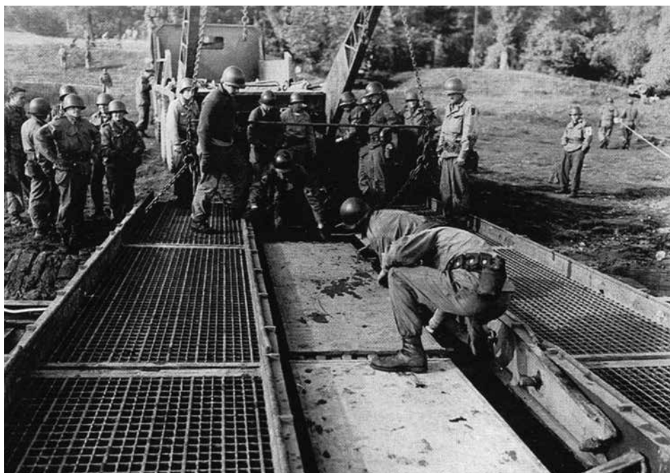
Engineers from Company A, 1st Engineer Battalion, build a ferry for the 1st Infantry Division during Exercise COMBINE.
